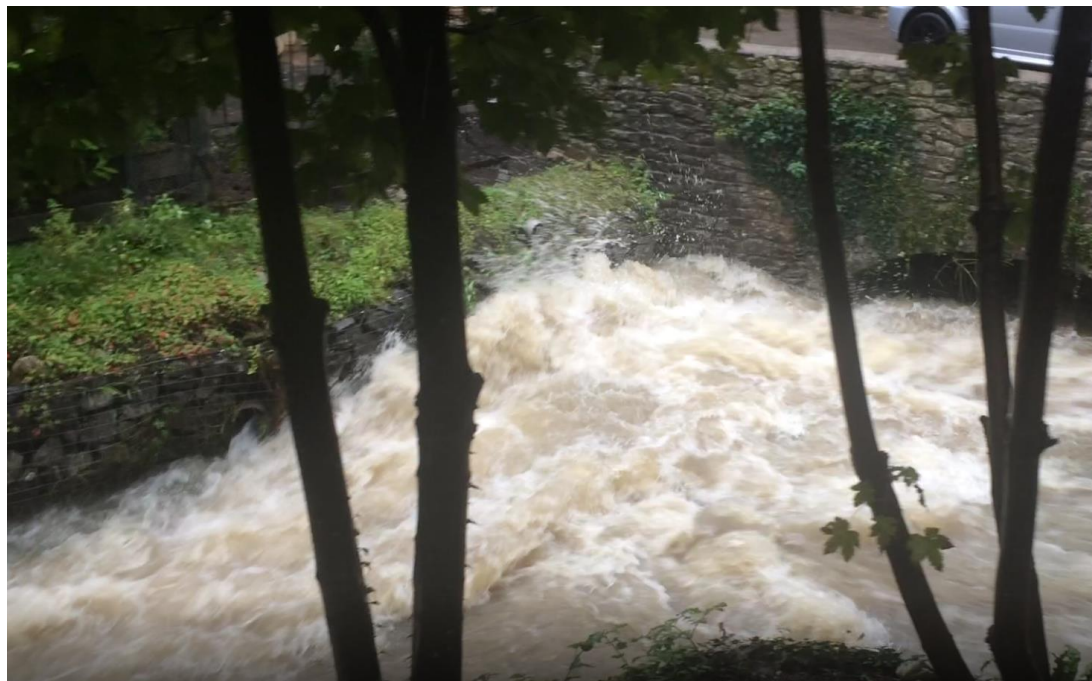
Figure 22 - Darshill Gabion Bank
